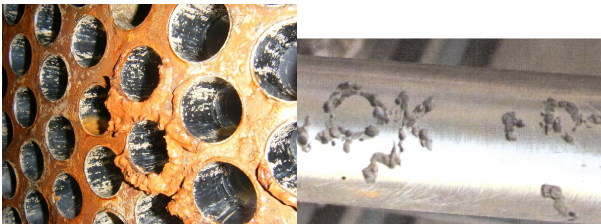
Figure 4. Two examples of unexpected crevice corrosion- the one on the left is of a 321 tube-to-tubesheet joint with S44660 tubes and that on the right is under paint in the shape of OK on a 416 stainless pump shaft
